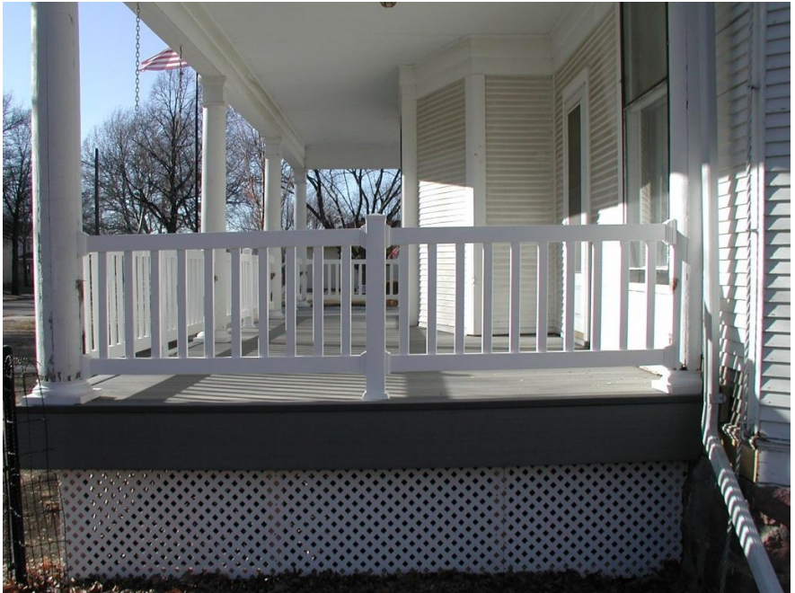
Above: The Completion of the Victorian porch project. See page 8 for full story.
