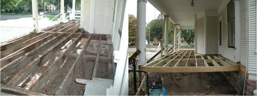
Left: Destruction phase is started. Right: Construction phase is under way.
